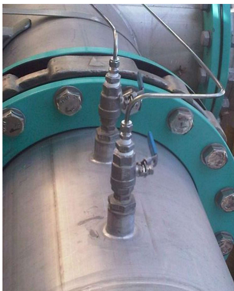
Figure 9 - Ball valve assembly
